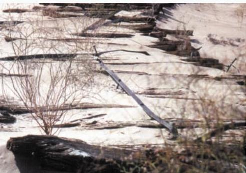
**Historic Plank Road –** Remnants of a "floating" wooden plank road that was used from 1916 to 1926 can still be seen in the Imperial Sand Dunes located on Gray's Well Road off Interstate 8 between Yuma and El Centro. (See additional Site Historic Marker description on page 33.) A small remnant is exhibited off Grays Well Road. Brochures are available at Buttercup Ranger Station. [desertusa.com/sandhills/planked.html](http://desertusa.com/sandhills/planked.html). Map Number 83.
